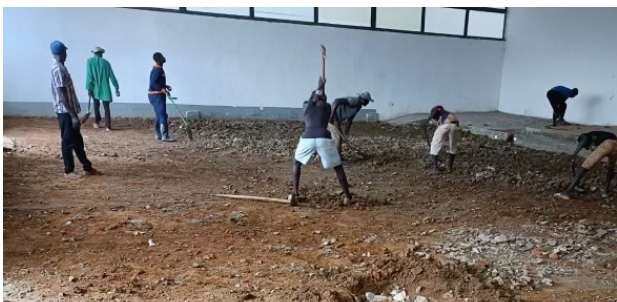
Removing old flooring
